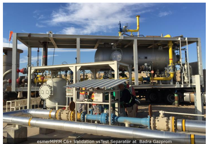
esmerMPFM C6+ Validation vs Test Separator at Badra Gazprom
